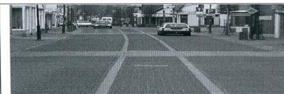
Access road: visual median in the centre of the village
